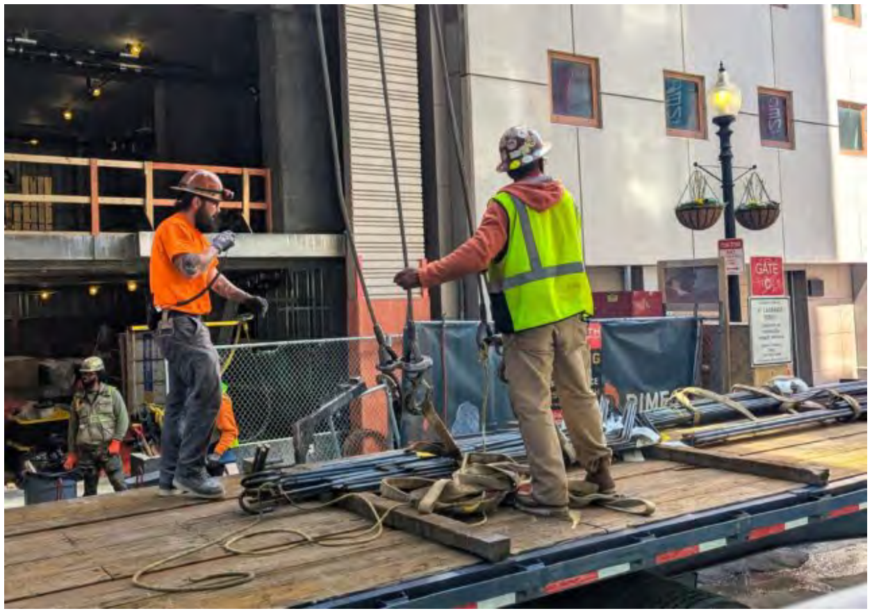
Construction workers prepare to lift rebar to the upper floors of the 41 LaGrange St. mixed-income housing development in Boston's Theater District in May 2025. Photo by James Sanna | Banker & Tradesman Staff
