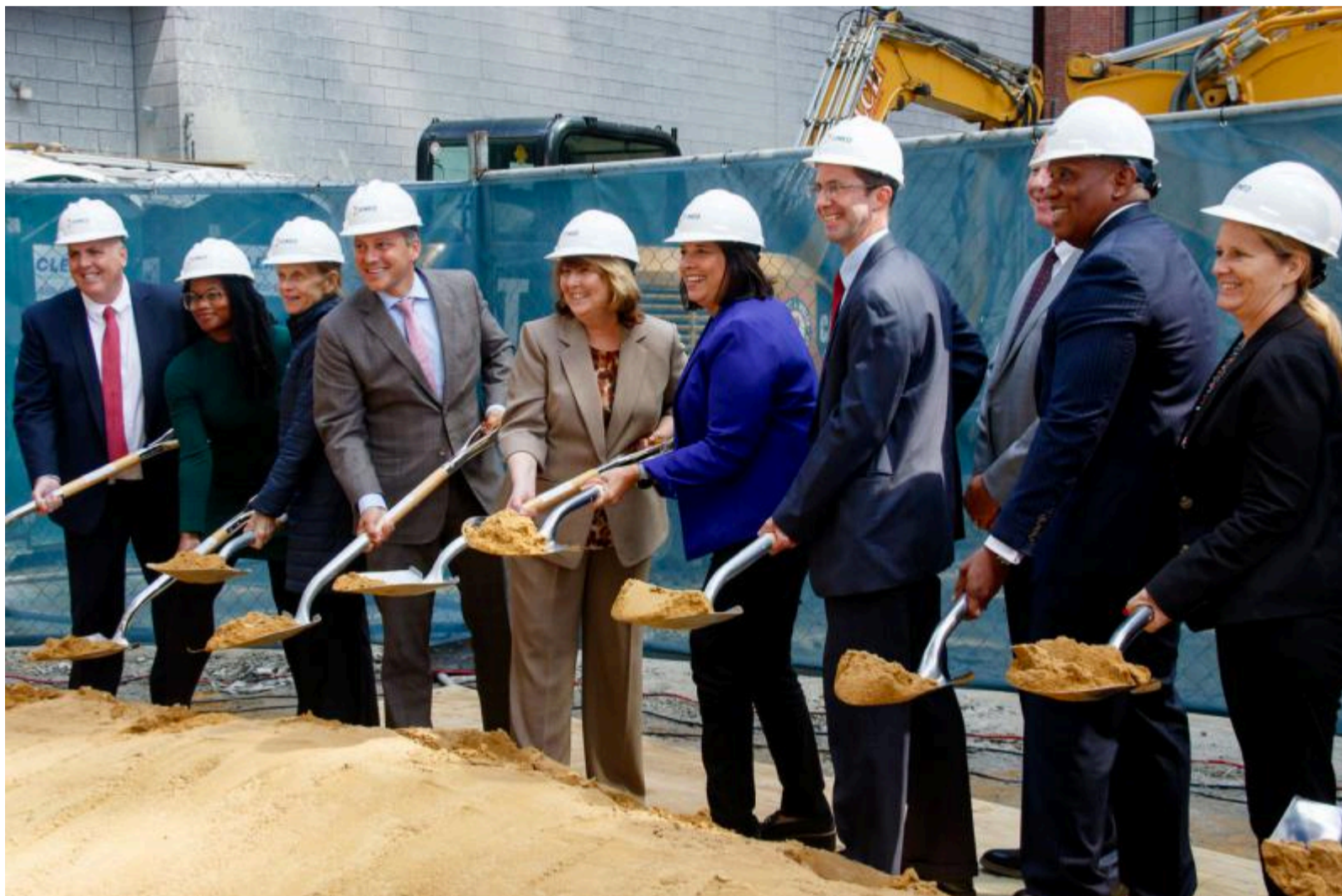
Lt. Gov. Kim Driscoll joins stakeholders and officials in breaking ground on the development at 41 LaGrange Street in downtown Boston. The 19-story, 126-unit mixed-income housing development is expected to be completed in 2026. Pilot photo/Wes Cipolla
